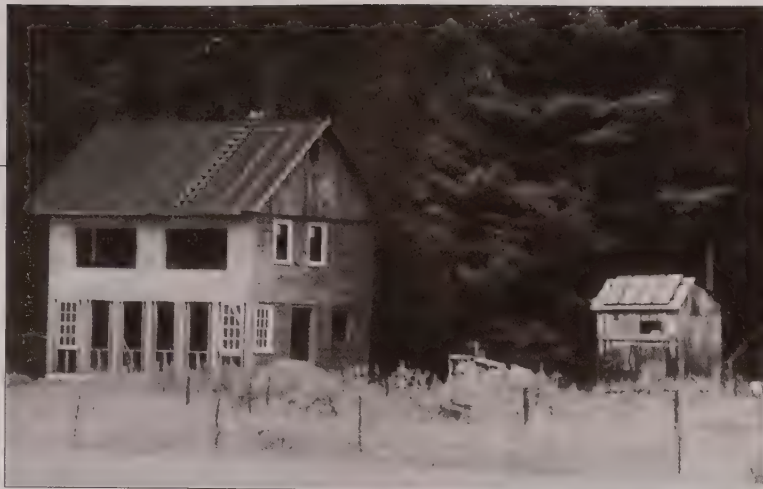
A house in a shaded location can utilize a "power shed" to position photovoltaic panels in the sun. Batteries and controls are close (for efficiency), snug, and safe inside.
